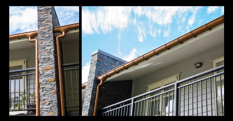
Spouting: Typhoon® Colour: Copper Bracket Type: External Downpipe: RP80® 80mm Round Downpipe Location: Ellerslie, Auckland
