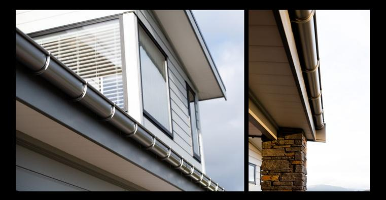
Spouting: Typhoon® Colour: Titanium Bracket Type: External Downpipe: RP80® 80mm Round Downpipe Location: Plimmerton, Porirua
