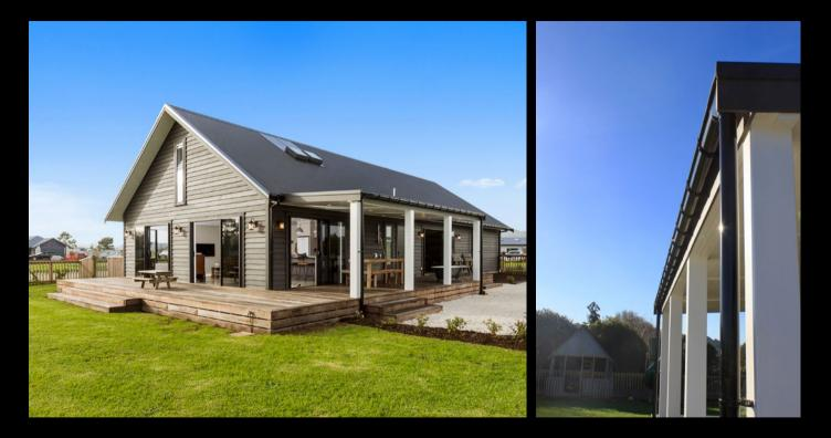
Spouting: Typhoon® Colour: Black Bracket Type: External Downpipe: RP80® 80mm Round Downpipe Location: Whitianga, Coromandel Peninsula
