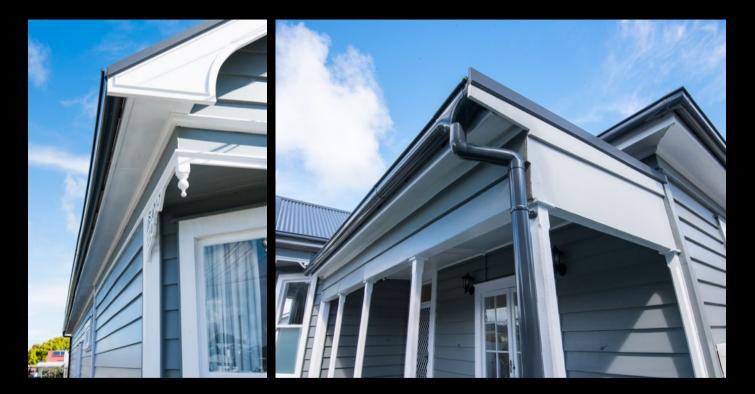
Spouting: Typhoon® Colour: Grey Friars® Bracket Type: Internal Downpipe: RP80® 80mm Round Downpipe Location: Sandringham, Auckland
