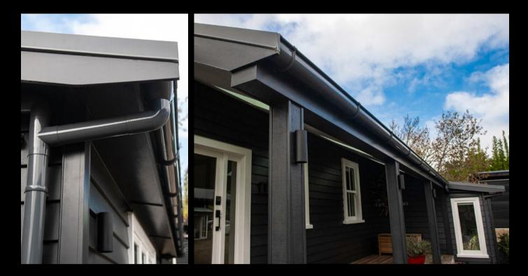
Spouting: Typhoon® Colour: Grey Friars® Bracket Type: Internal and External Downpipe: RP80® 80mm Round Downpipe Location: Dairy Flat, Auckland
