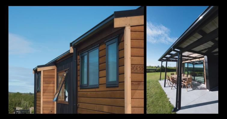
Spouting: Typhoon® Colour: Black Bracket Type: Internal Downpipe: RP80® 80mm Round Downpipe Location: Hawera, Taranaki
