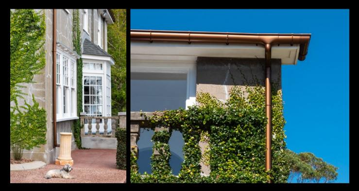
Spouting: Typhoon® Colour: Copper Bracket Type: External Downpipe: RP80® 80mm Round Downpipe Location: Clevdon, Auckland
