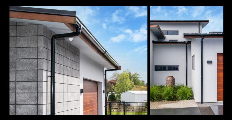
Spouting: Typhoon® Colour: Black Bracket Type: Internal Downpipe: RP80® 80mm Round Downpipe Location: Stratford, Taranaki
